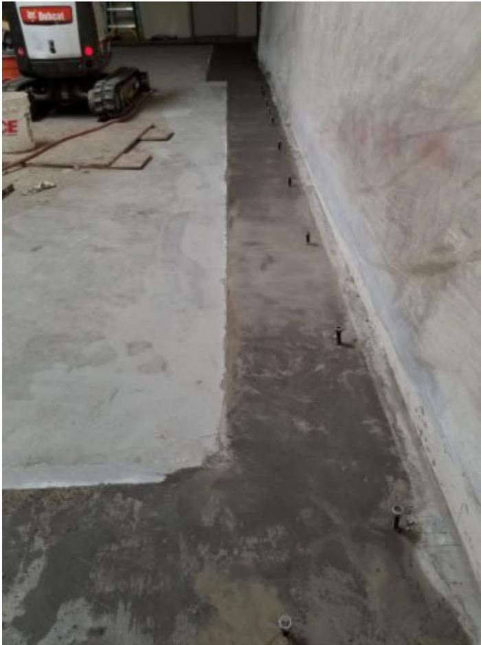
The foundation has been poured and leveled. Note the anchor bolts have been positioned and are now standing proud. Watch your step! PHOTO: Bruce Black
