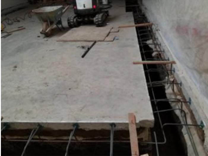
The trench is dug and the rebar is installed; waiting for the anchor bolts and the pour. Note how close the trench is to the industrial unit's boundary wall. PHOTO: Bruce Black
